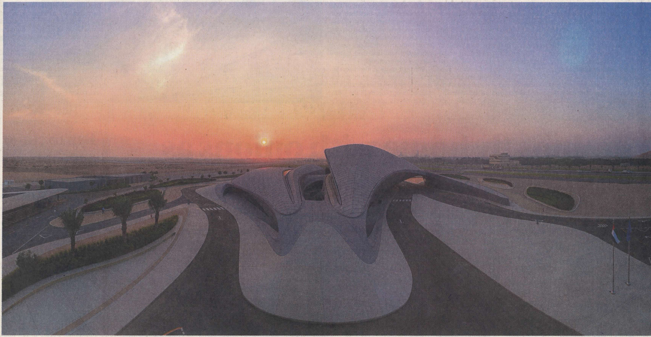
The BEAAH Group's ground-breaking new headquarters building, designed by Zaha Hadid Architects, has been imagined as an "Office of the Future", with sustainability and digitalisation as its core principles. — SUPPLIED PHOTO
